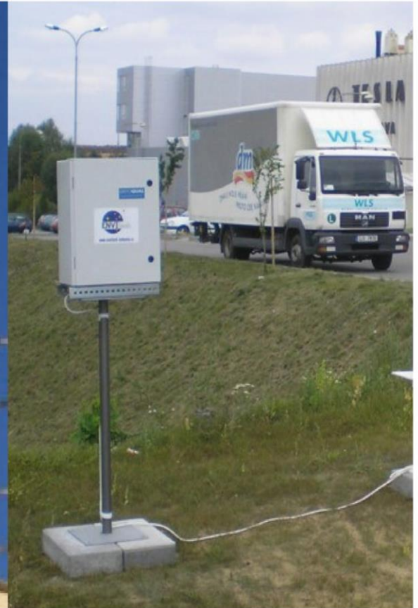
Roadside and traffic monitoring
